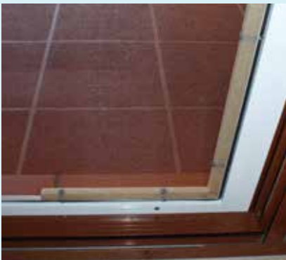
Bracket fitted - inside view
