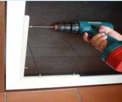
Bracket being fitted - outside view
